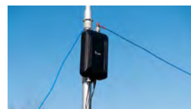
Wire antenna installation example
